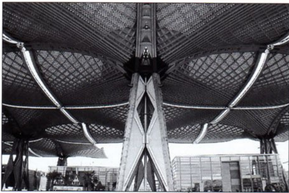
Fig. 5: Roof structure for Expo World Exhibition in 2000 in Hanover constructed with stacked planks
